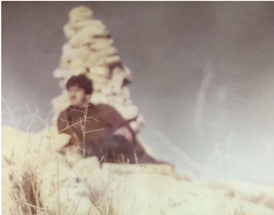
Figure 6. Shows the stone cone, which is made of stacked stones without using any binding material.
